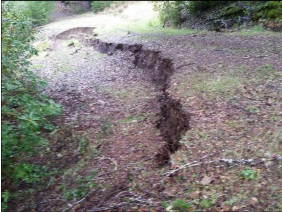
Photo 9a: Site #48.1, looking at the failing outboard edge of fill from left road.
