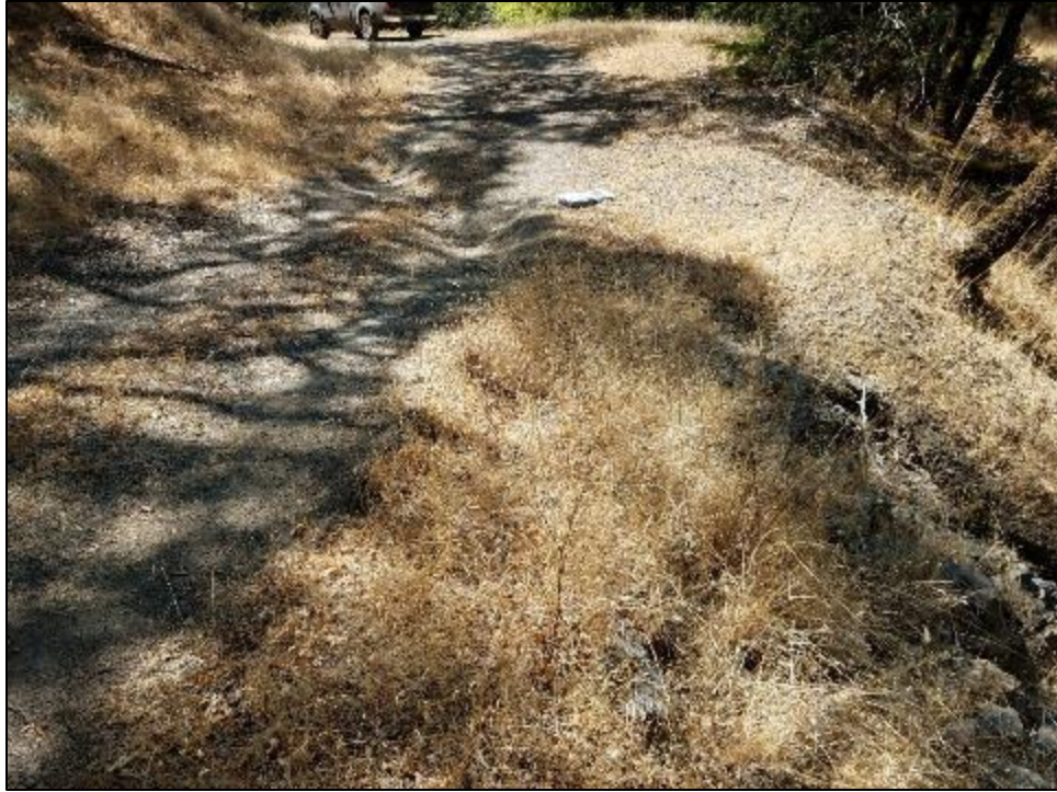
Photo 4a: Rolling Dip #62, looking up the road from the outboard edge of road fill.
