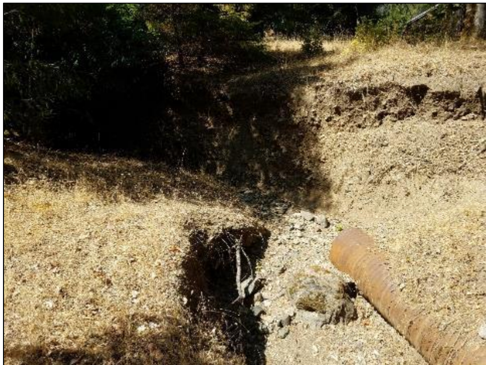
Photo 10b: Site #30.9, looking upstream at washed-out stream crossing and vertical banks.
