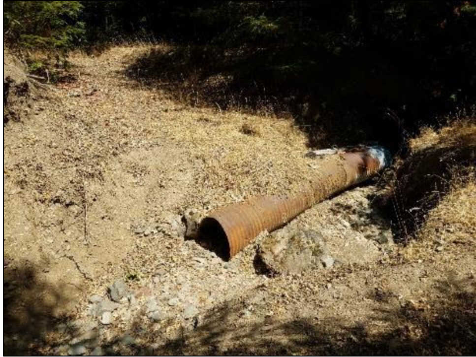
Photo 10a: Site #30.9, looking downstream at washed-out stream crossing and left bank.
